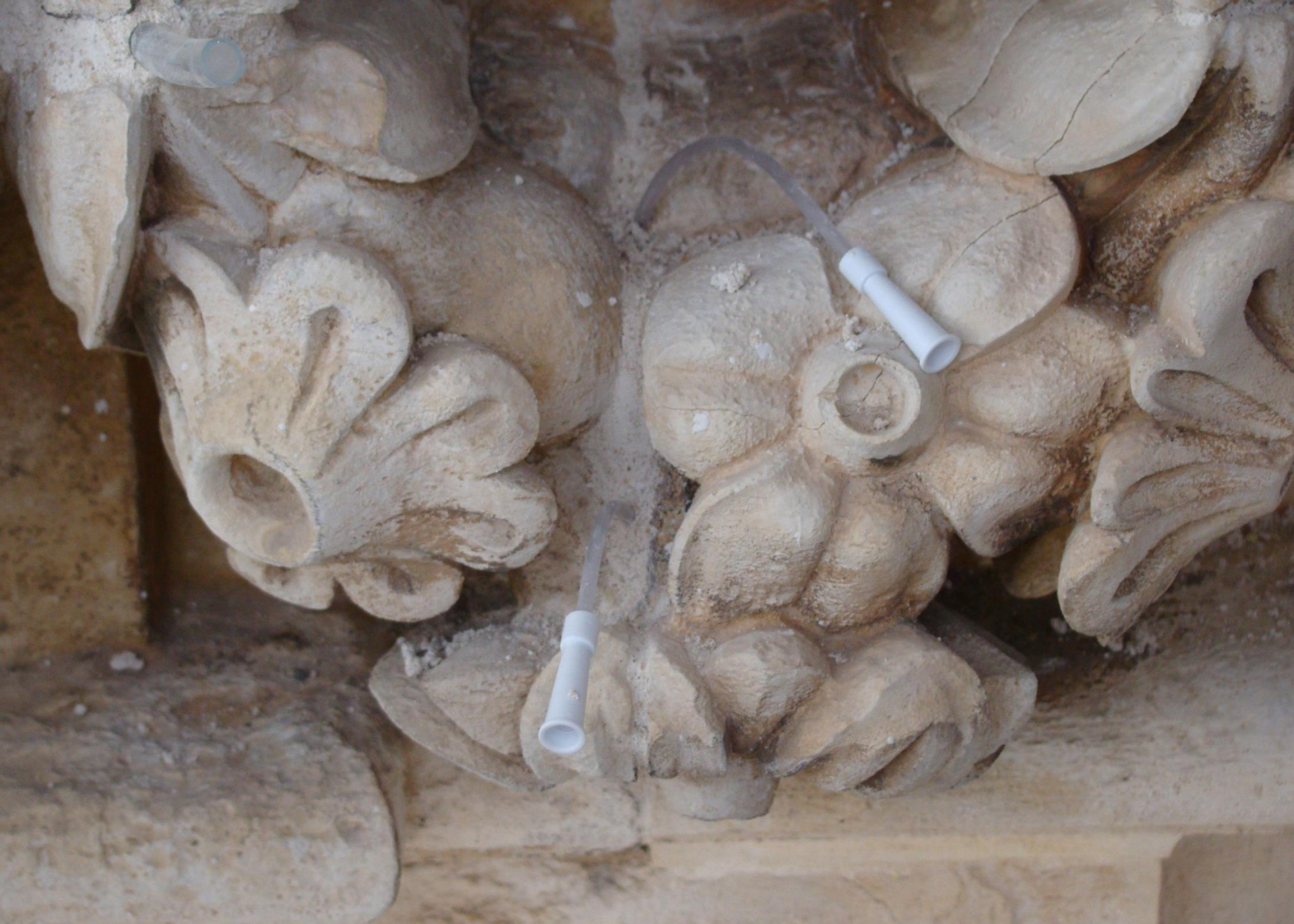
University Tower | Conservation and Restoration Works | 2012
