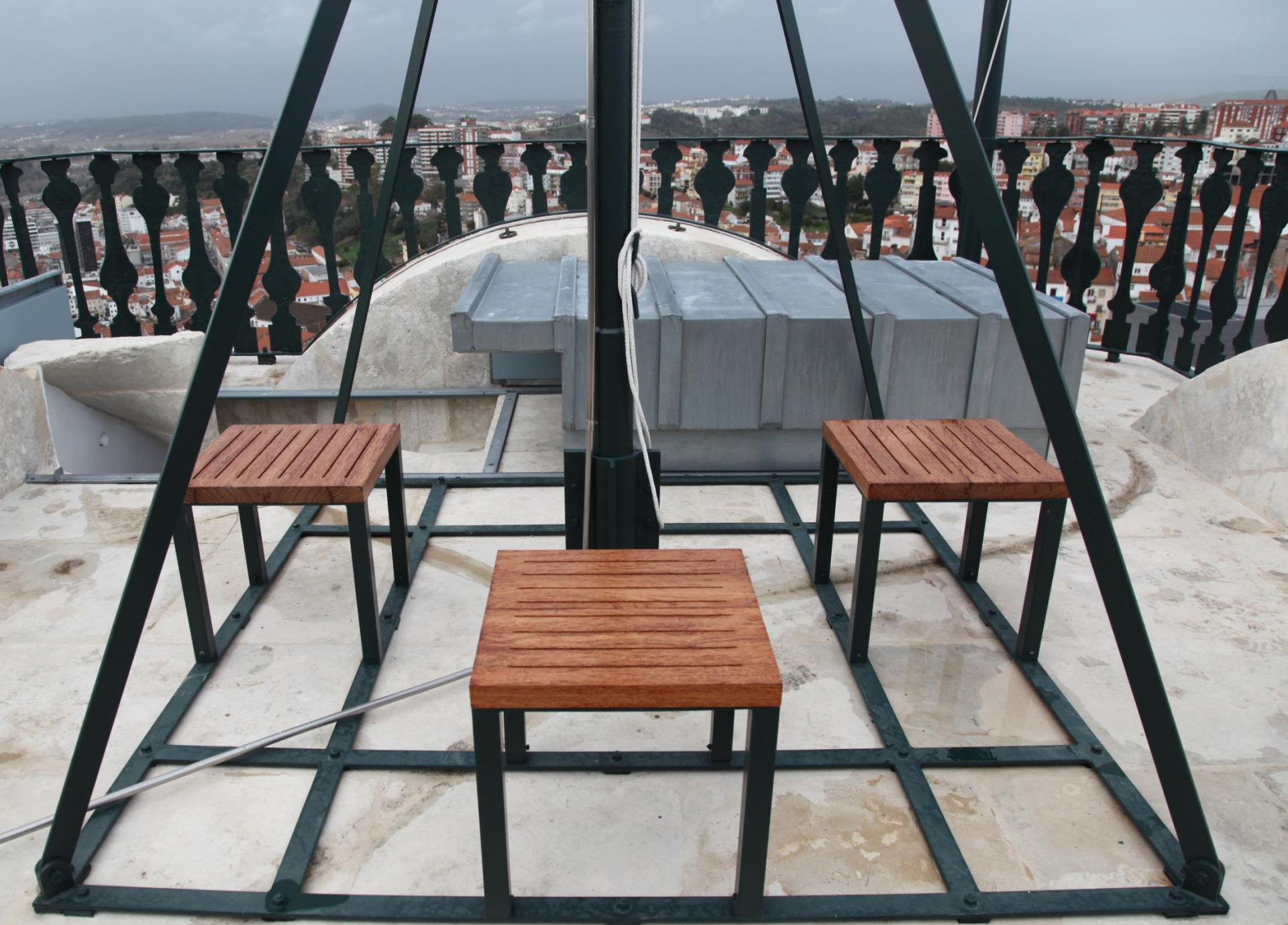
University Tower | Conservation and Restoration Works | 2012
