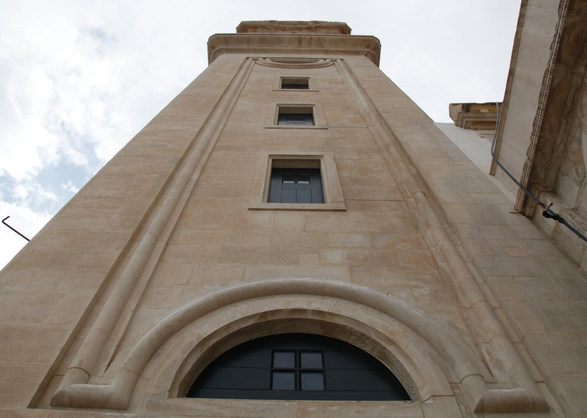
University Tower | Conservation and Restoration Works | 2012
