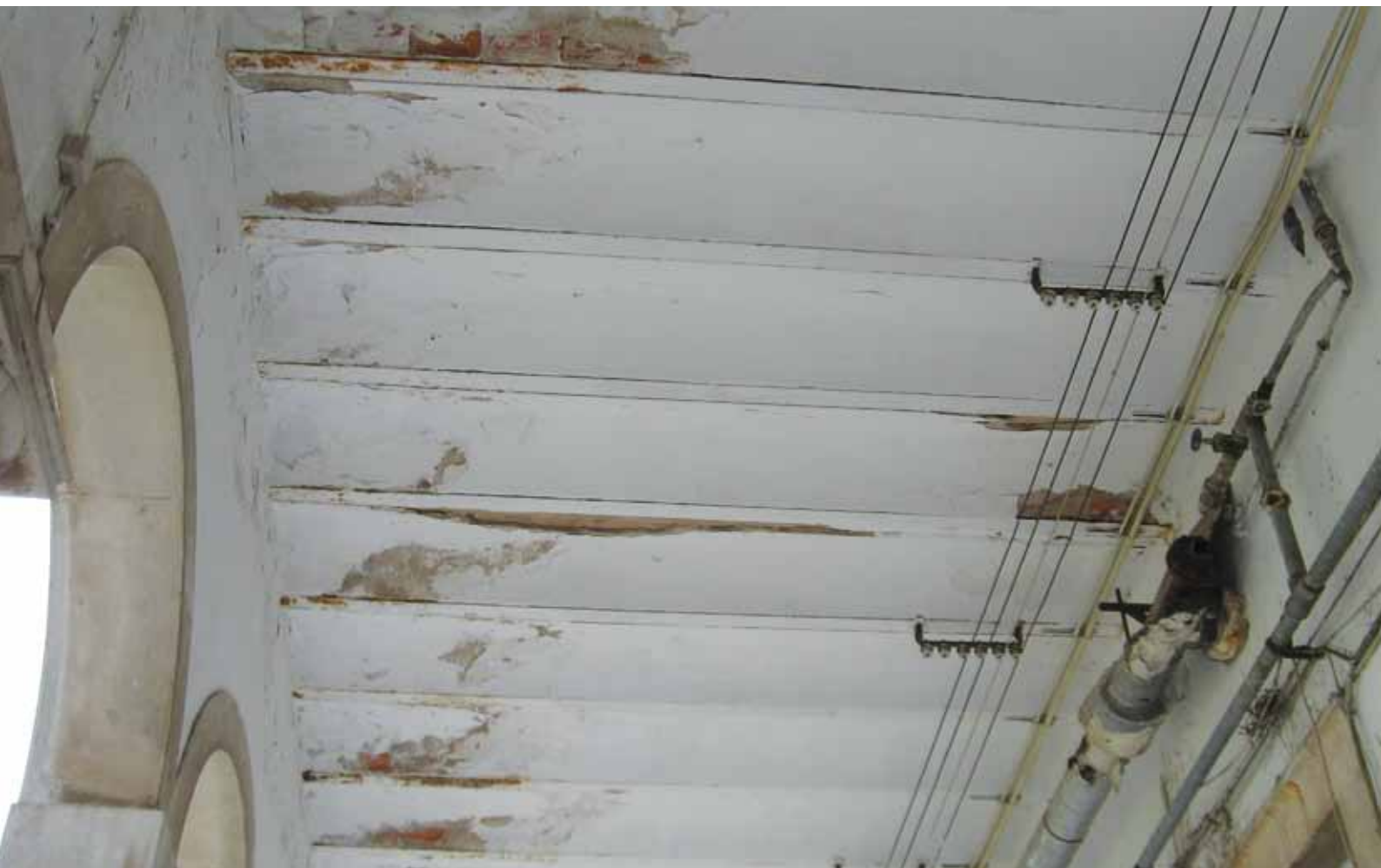
Deterioração do tecto no piso inferior do claustro do Colégio das Artes, SSR, 2008 Deterioration of ceiling on the lower floor of the cloister of the College of Arts, SSR, 2008
